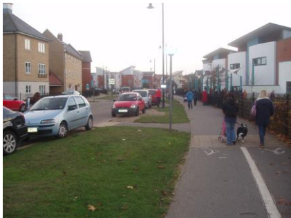
Poor design consideration to the grass verge outside the school with inevitable results. Parking could be within School playground as Milton Keynes?
