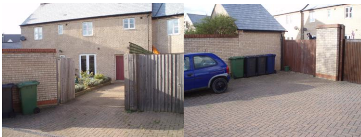
Some housing rear access to rear gardens for car parking and garages tended to be blocked by bins and other parked cars
