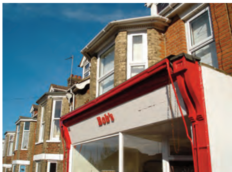
Traditional shopfront, Felixstowe Road. These should be retained and restored wherever possible
